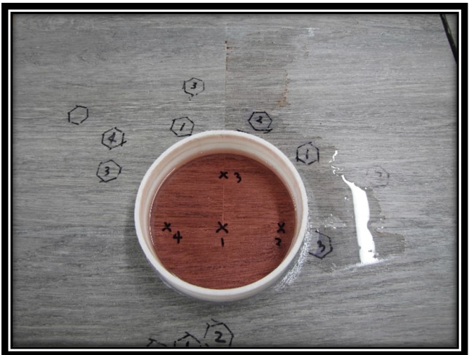
Water was able to channel through the joints and puddle on the surface of the planks.
