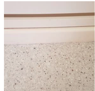
After fitted any excess silicone that squeezes up is removed
