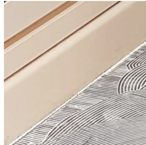
Silicone to the shower/ floor junction
