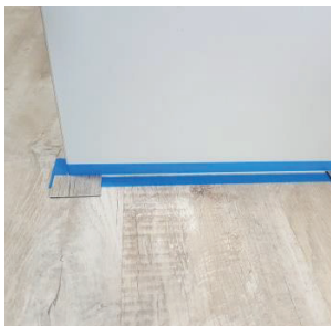
Setting the bead width
